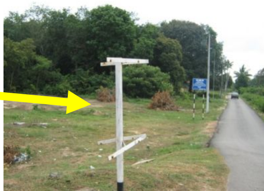
Gambar 1.10 Chevron Delineator Hilang
