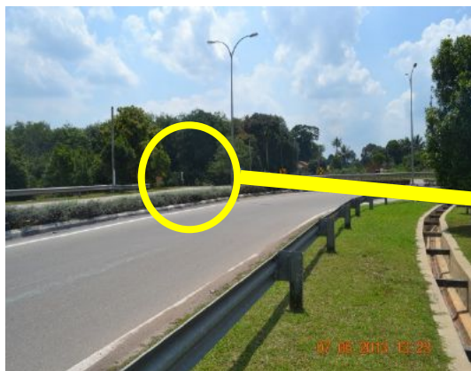
Gambar 1.10 Chevron Delineator Hilang
